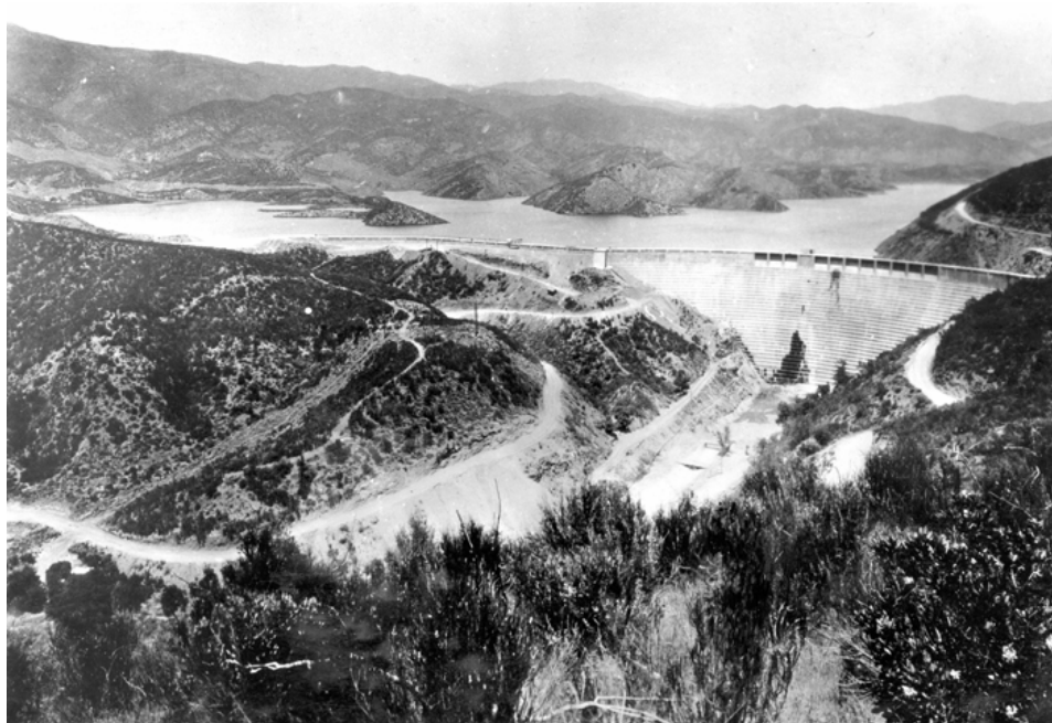
St. Francis Dam
